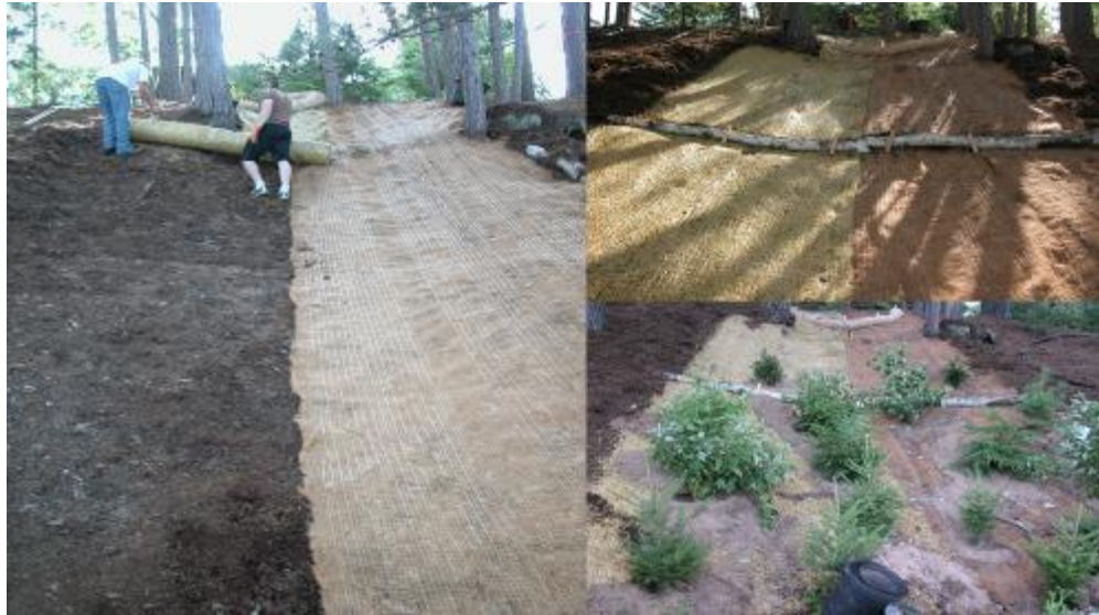
Figure 24 Installation of erosion control blankets in the summer of 2011 on Mirek's Property, LSG Lake. Two types of blankets were used, coconut coir and straw
