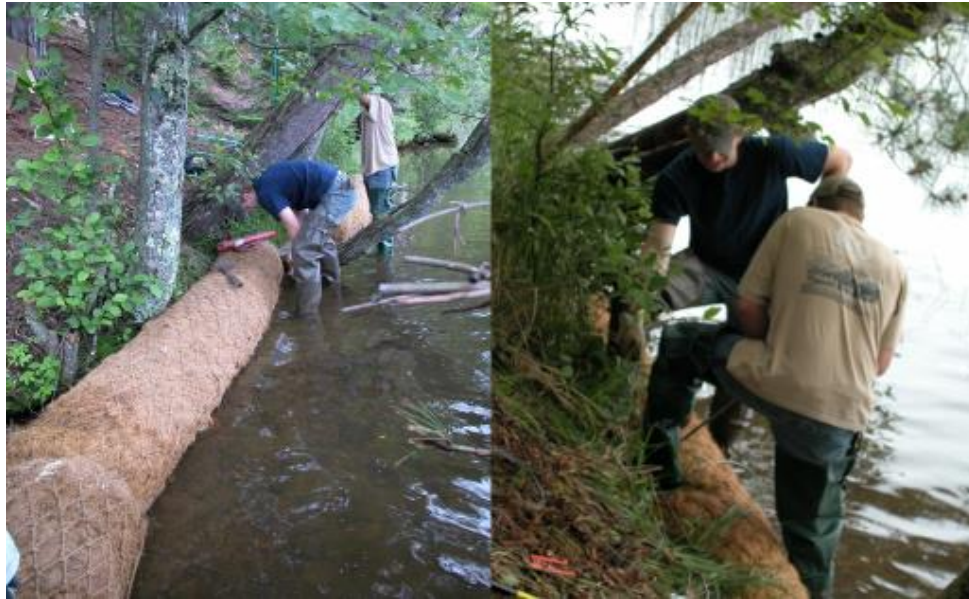
Figure 26 Installation of biologs at BJW-SP property on LSG in June 2011. Biologs were secured to the lake bed using cabled earth anchors and then planted with native wetland plants.
