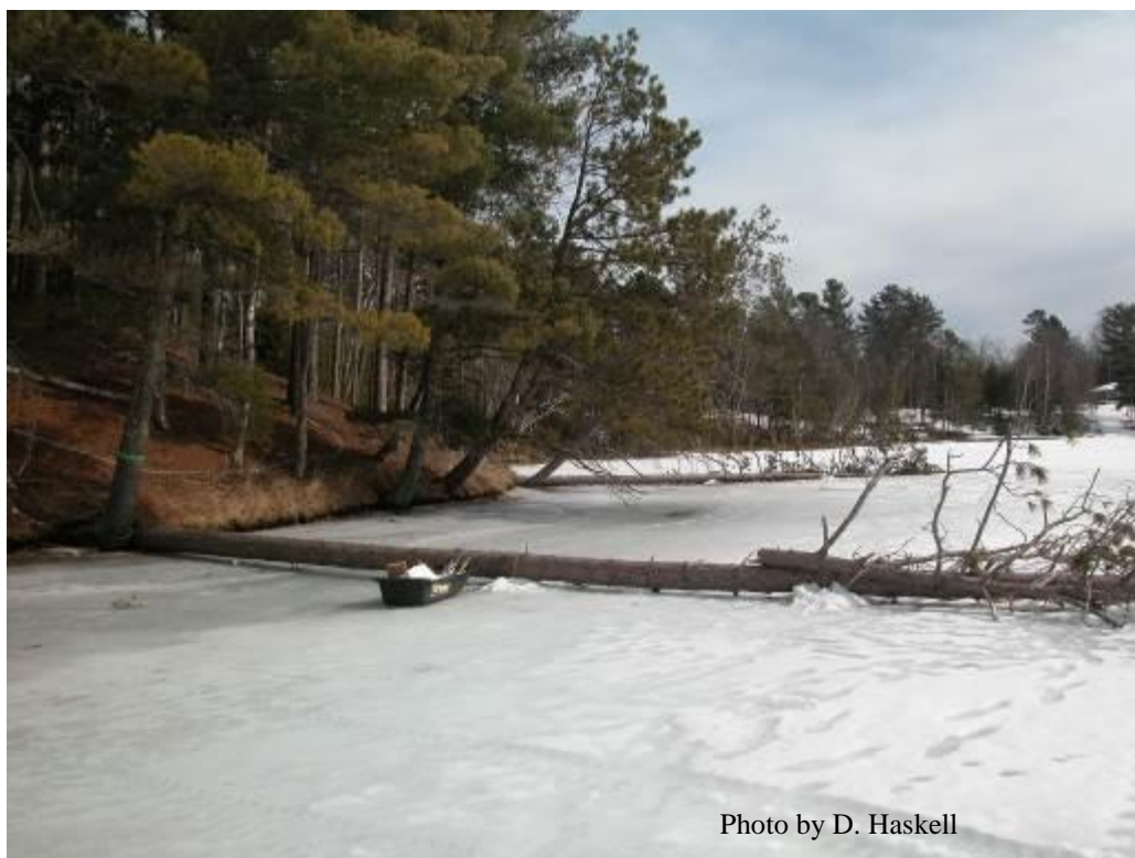
Figure 27 Tree drops installed at Lou Mirek's Property on LSG Lake during the winter of 2011. Trees were later secured to lake bed using steel cables and earth anchors.
